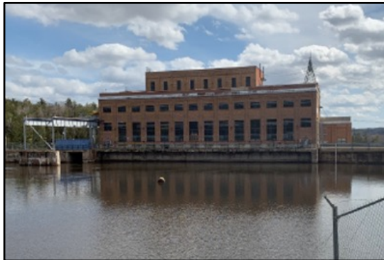
Heavy turbine leakage was causing issues.
